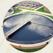
Water treatment Plant
