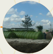
Sewage Treatment Plant
